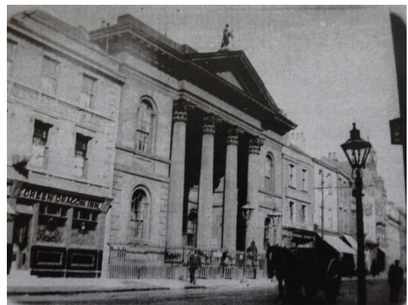
The Guildhall, Frenchgate, Doncaster, 1847 (Courtesy of Heritage Doncaster)
